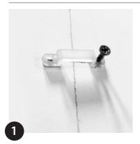
Mark and drill (if required) for screws. Fix clips with 1 suitable screw (min. 5 clips per metre or every 250mm/9.84").
