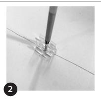
Fix clips with suitable screws.
