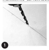
Mark and drill (if required) for screws (min. 5 clips per metre or every 250mm/9.84").
